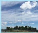
High Island, New York (Transmission Antenna)
